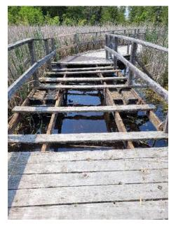
Work on the Marsh boardwalk continues. Scheduled maintenance was complicated by the vandalism, increasing the amount of work required. Supports and struts needed to be replaced, and new deck boards installed. We anticipate these repairs will be completed by the end of July. In addition to fixing the damages, we are replacing materials with plastic wood to increase the longevity of this infrastructure.
